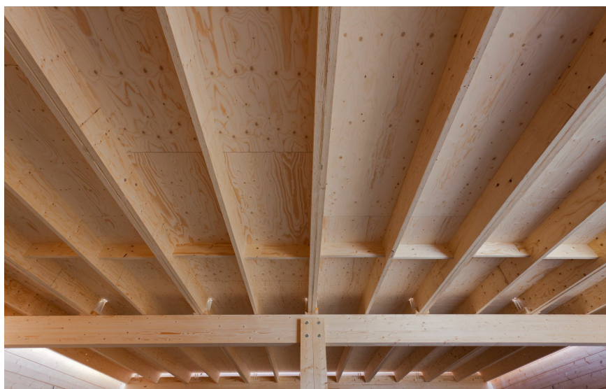
Metsa Kerto LVL, in-build application.
