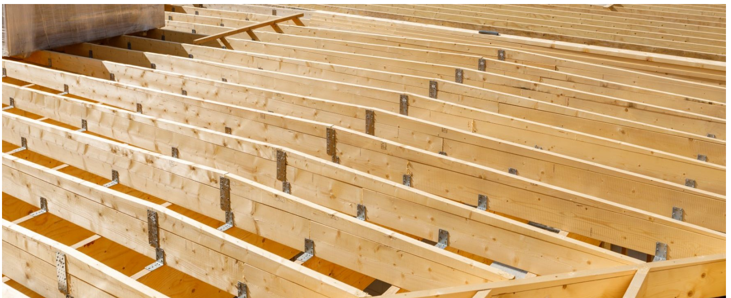
Metsa Kerto LVL, rafters in-build application.
