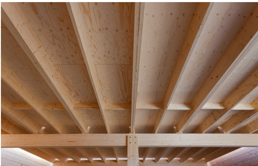
Metsa Kerto LVL, in-build application.
