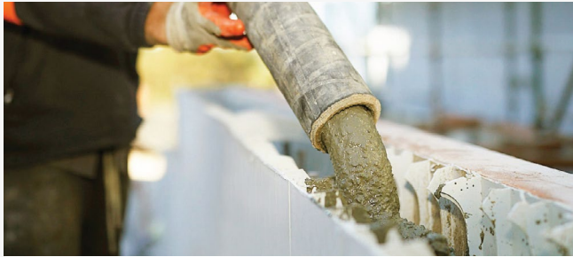
Step 6 Core filling.
